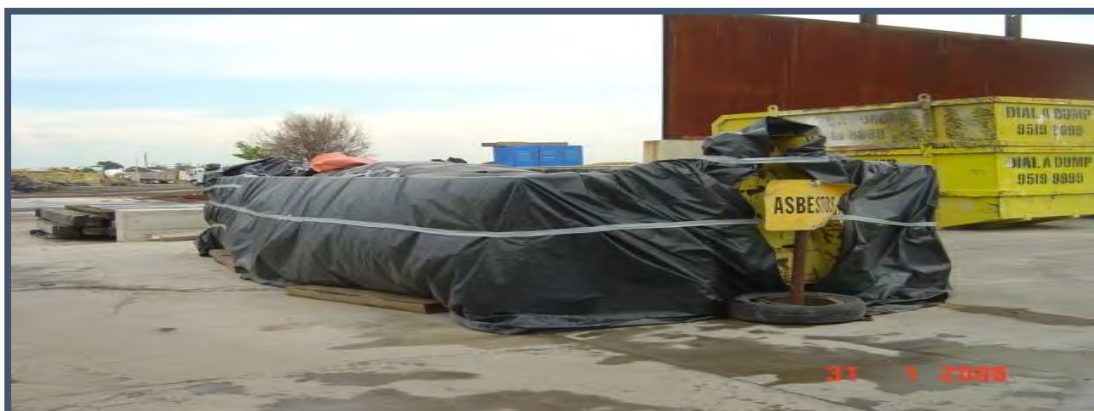
Fully covered hook bins can be used to store ACM in the Designed Clean Areas
