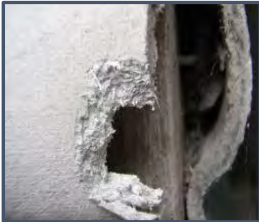
Fibro Sheeting (By m3)
