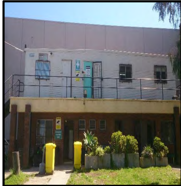
Site Office at Alexandria
