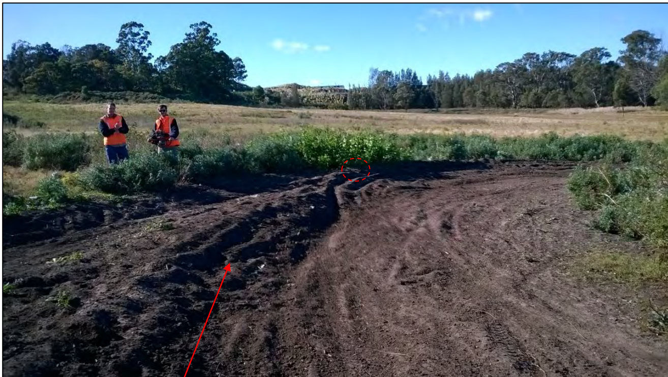
Photograph 4. Subject site, fill materials
